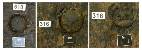
These treenails are around 300mm long and a consistent 30mm in diameter, and there were about 8,000 of them used in our Ship. Treenails were commonly used in timber framing both for ships and houses but ours are unique in one respect: rather than being roughly carved on a shaving horse, many of them have been turned on a lathe, at least for their upper length, so that they fit exactly into the augur holes in the frames.
